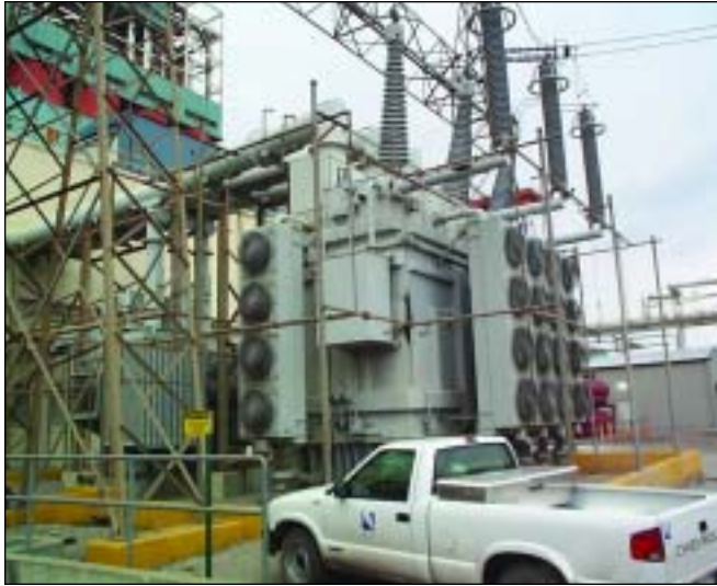
Transformers and related equipment often require protection from moderate exterior exposures.
