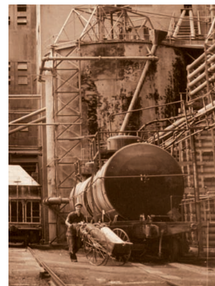
(Above) Franklin Strain (standing) was the co-developer of allyl diglycol carbonate (CR-39 monomer) along with Frank Muskat. (Right) Sitting in PPG's Barberton, OH, shipping yard in 1945, this railroad tank car filled with 38,000 pounds of CR-39 monomer prompted the search for civilian uses for allyl diglycol carbonate and the development of lightweight plastic ophthalmic lenses.
