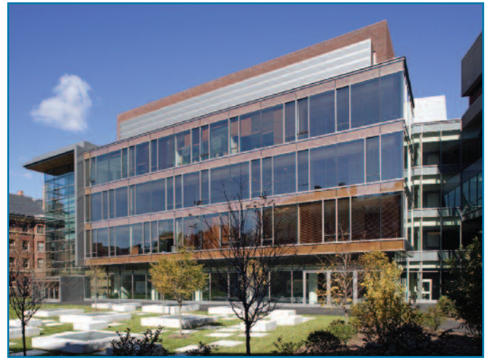
Solarban 70XL glass provides maximum daylight and excellent solar control, mitigating the need for artificial lighting and cooling.
