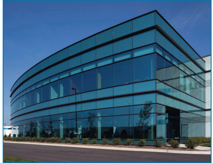
Vistacool Azuria glass combines with Sungate 500 glass to create energy savings as well as a lustrous aqua-blue sheen for the Bolingbrook, IL based glazing contractor, Frontrunner Glass & Metals.
